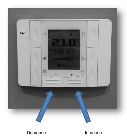
This control only allows the air conditioning unit to increase or decrease the temperature inside the Lecture Theatre manually by 5 degrees each way from pre-set 21°C.
